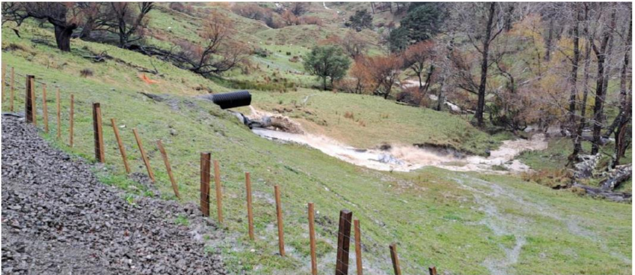
Figure above is existing waterflow from the TREC Culvert underslip work programmed planned
