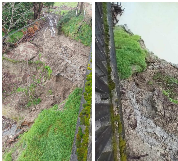
Pictures of these two figures above taken from different angles of the banks around the pilings of the bridge at the same time as the previous photo – J Symes approximately 2 weeks after Cyclone Gabrielle
